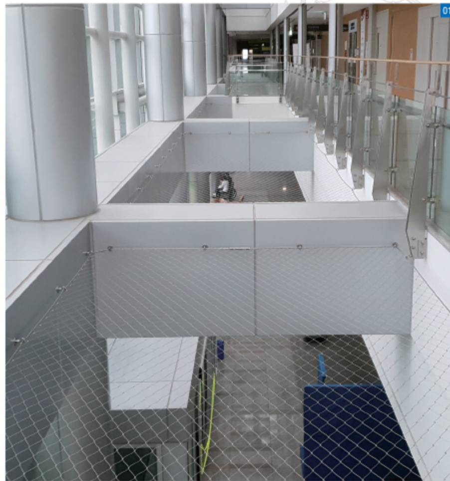
01 제주대학병원 Jeju National University Hospital 웹넷 추락방지 안전망 Webnet fall protection safety net
